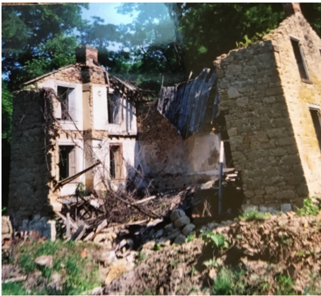
House at the start of the project in 2006.
